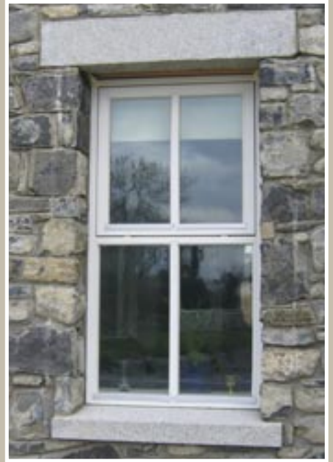
Granite lintel Length x 200 x 250mm
