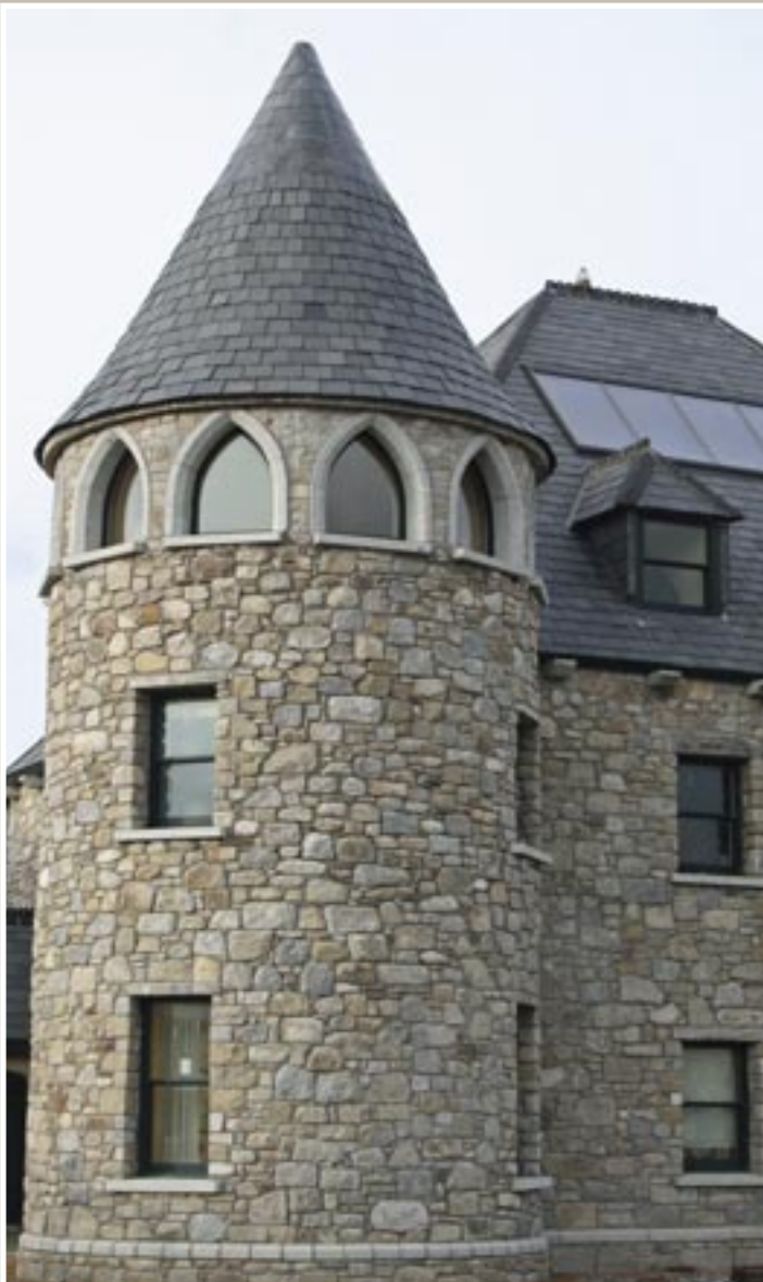
Granite lintel Length x 215 x 100mm Length x 135 x 100mm
