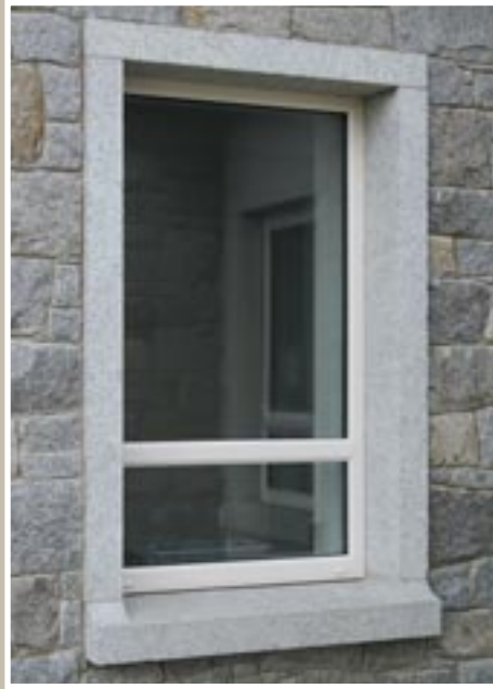
Granite lintel Length x 215 x 100mm Length x 135 x 100mm
